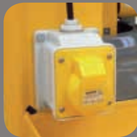
AC power to platform
